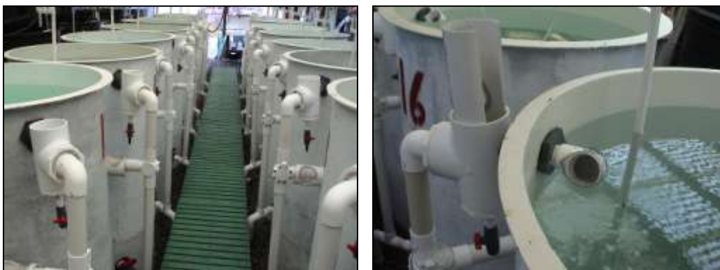
Figure 1. Replicated (19 tank) marine ornamental broodstock holding system with surface egg collector system for gentle collection of small floating eggs from pelagic spawning reef species such as the flame angelfish.
