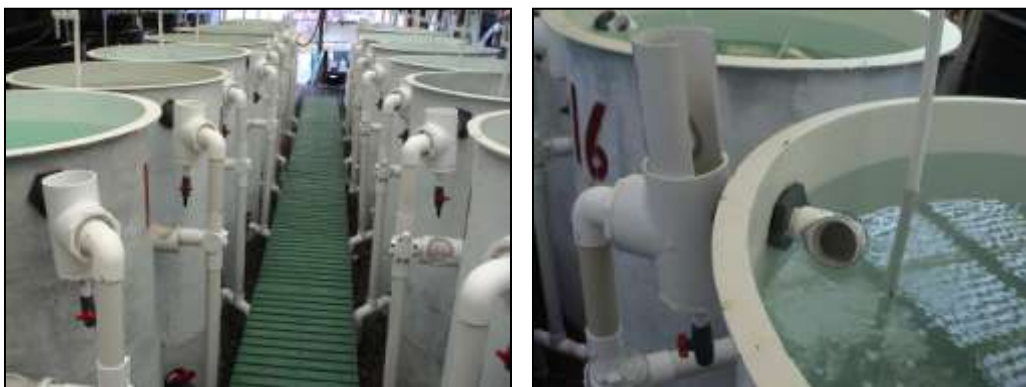
Figure 1. Replicated (19 tank) marine ornamental broodstock holding system with surface egg collector system for gentle collection of small floating eggs from pelagic spawning reef species such as the flame angelfish.
